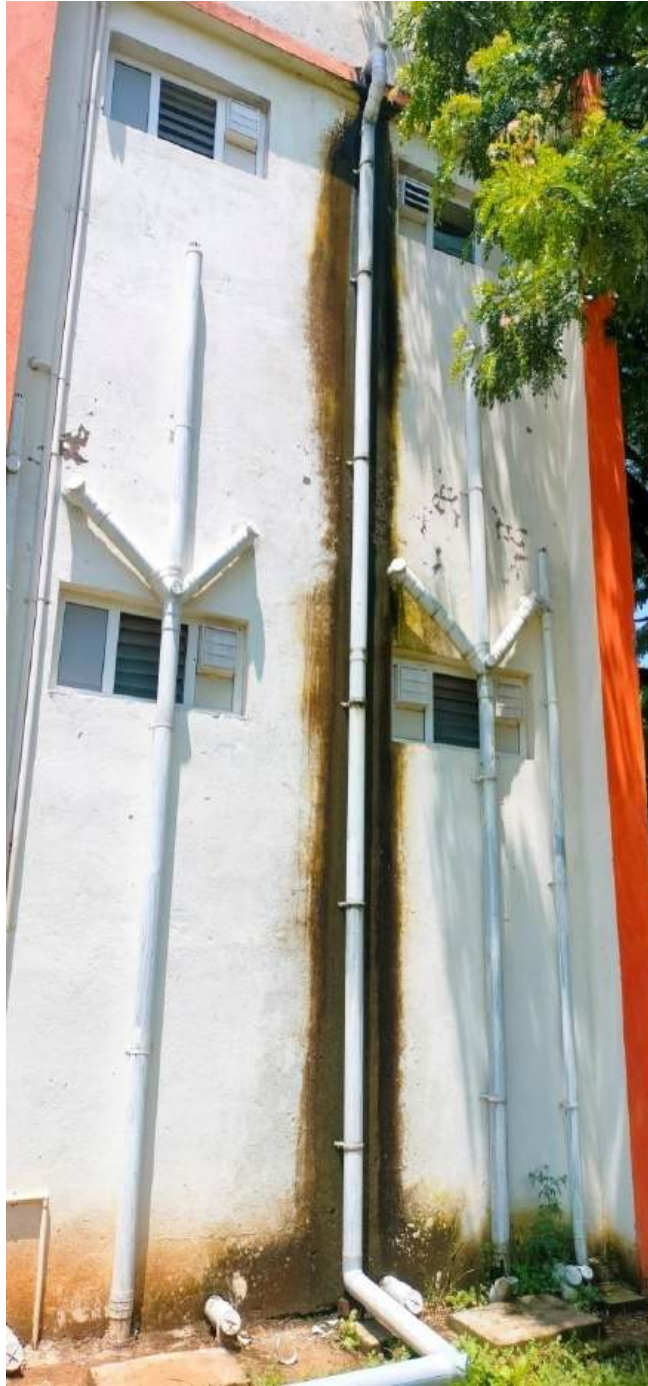
Pipe Line connecting roof area to water storing tank.
