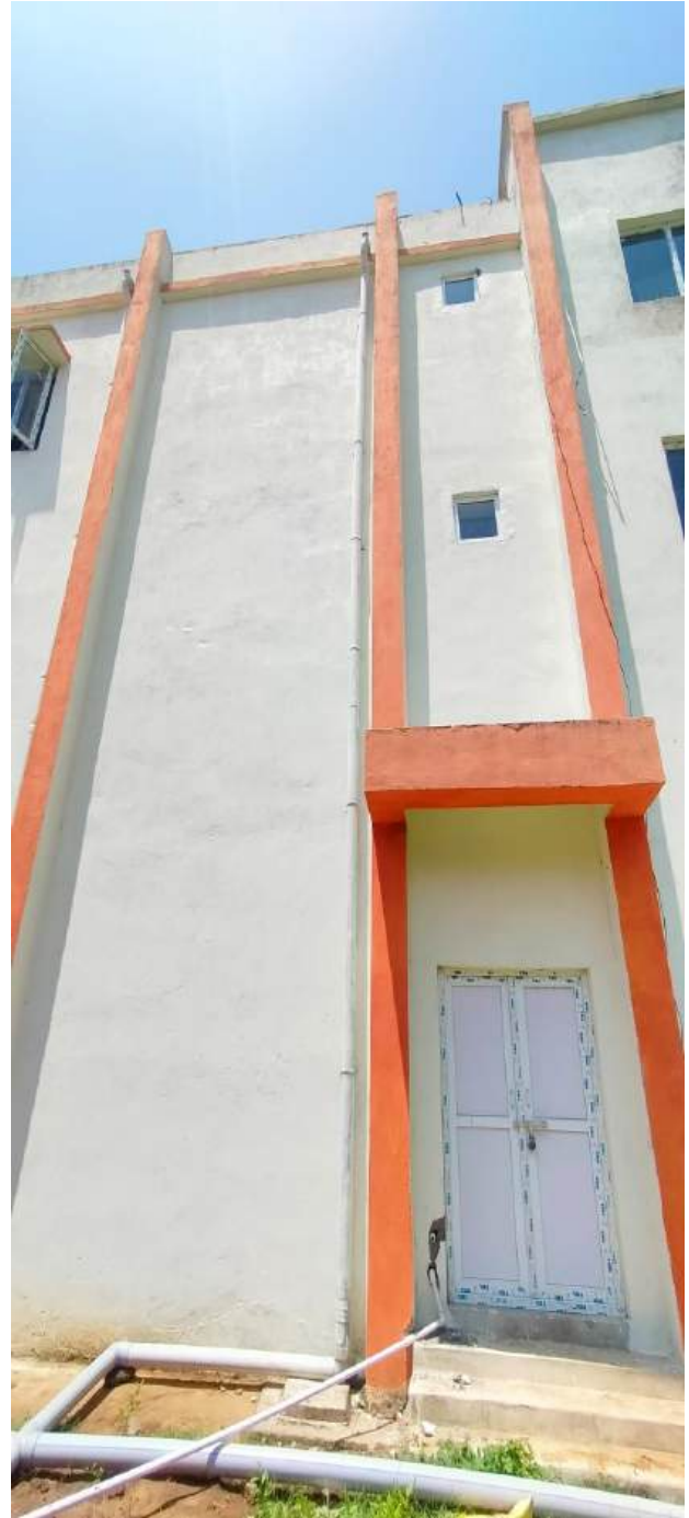
Pipe Line connecting roof area to water storing tank.
